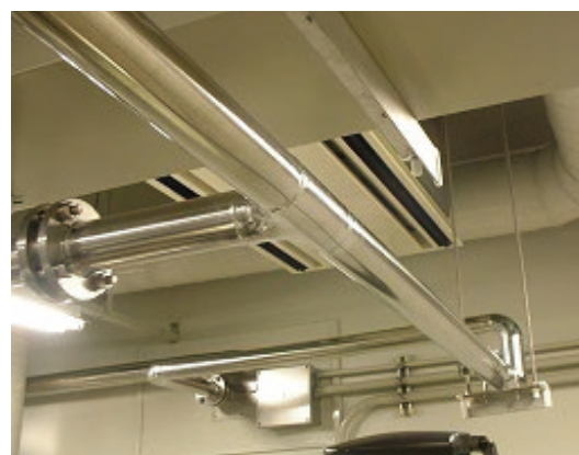
Vacuum-insulated pipe.
